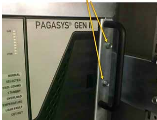
Figure 65 Removing the chassis mounting screws
