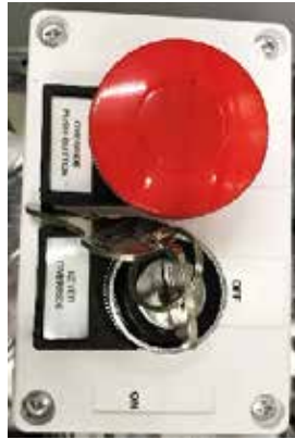
Figure 70 Lower/Raise siren head rotating switch
