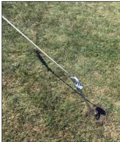
Figure 68 Cable attached to the ground anchor
