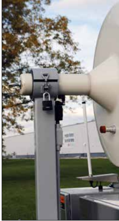
Figure 77 Siren head with lock
