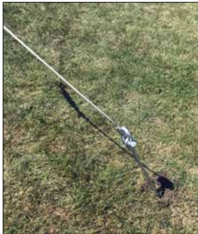
Figure 60 Cable attached to the ground anchor
