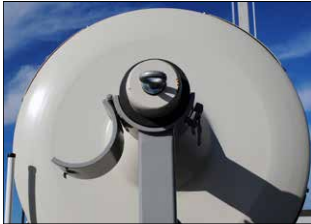
Figure 49 Siren with unlatched siren restraint
